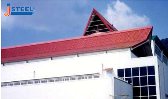
Wayang Windu Power Plant - Bandung
